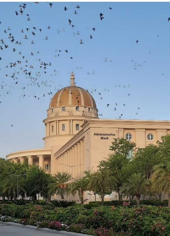
Administrative building of MUJ with the International and the IAESTE office, library, offices, and conference rooms.
